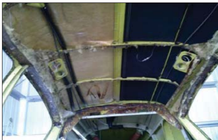
Removing the old panels and insulation.
